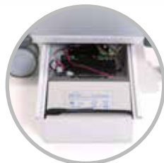
6. Power Pack including battery and controller
