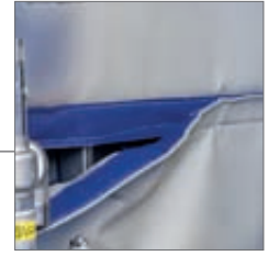
Heat insulation with durable fabric covering for improved service maintenance
